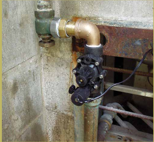
Before and after I-CON System's Momentum Flush Valve installation that seals with minimum water pressure, preventing potential flooding scenarios.
